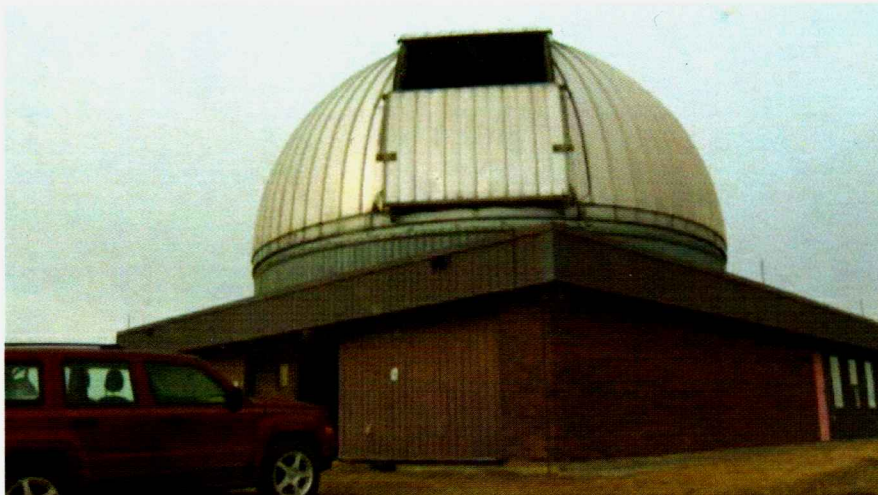
The Rothney Observatory may have difficulty looking at the night sky due to light from the ring road.
